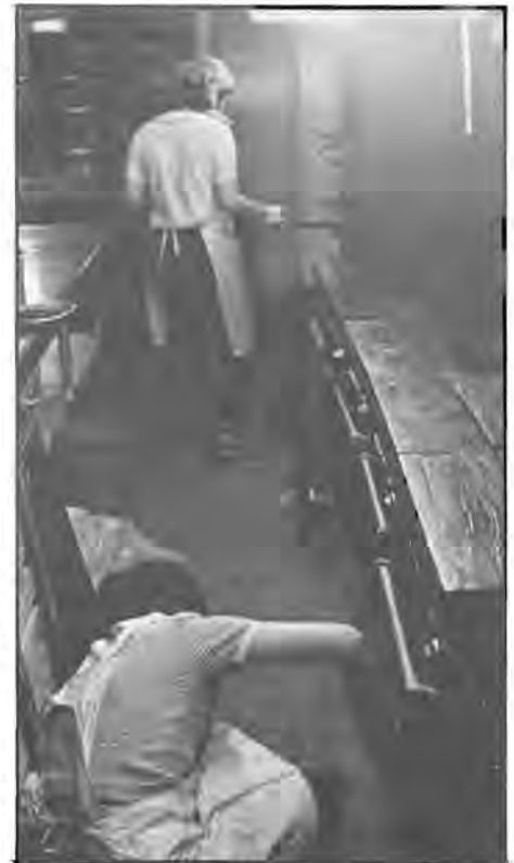
Many people worked on the cooking area of the large basement kitchen. (Right) Naval Jelly removes rust from the stove as work continues.
