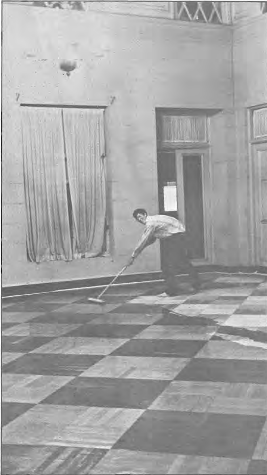
Dennis Taylor applying polyurethane protector to ballroom floor.
