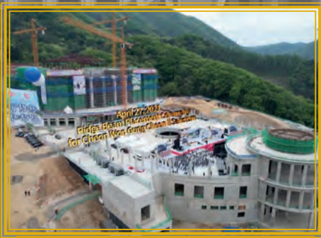
Ridge Beam Placement, April 2021
