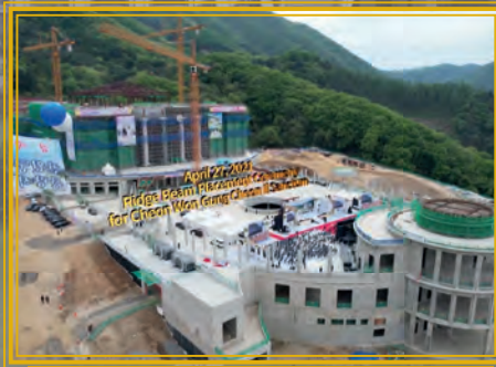
Ridge Beam Placement, April 2021
