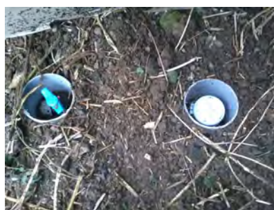
New sub water meter installed
