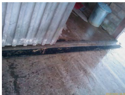
A drain has been put in front of stables on South Farm where water was flooding the stables.
