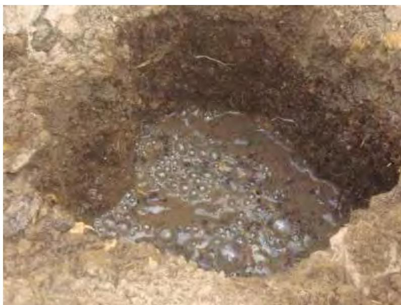
Not to be deterred, several volunteers jumped back into the holes and filled buckets with water and wet soil. Water seepage was not going to stop them! Yet, despite their best efforts, it did not take long for the volume of muddy soil removed to be replaced by an equal volume of water. Frustration was growing because we needed to dig wide holes to the depth of eight feet as a foundation to install a hand drill.
