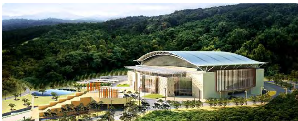
Cheongshim Peace World Center under Construction.
