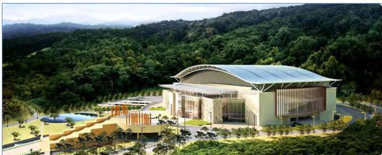
Cheongshim Peace World Center under Construction
