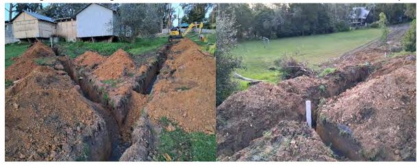
Pipes have been laid and signed off up to the toilet block, the next step is to empty the septic tanks and connect the pipes to the sewerage line. Special care was taken to add side pipes for future toilets.
