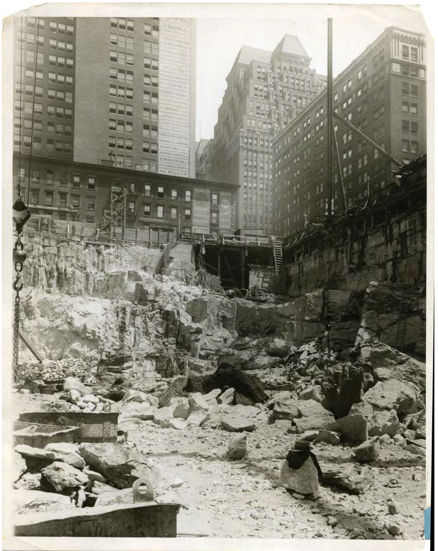
Over 2 million cubic feet of solid rock was excavated on the corner of 34th and 8th. The hotel was set to be 75 feet deep.
