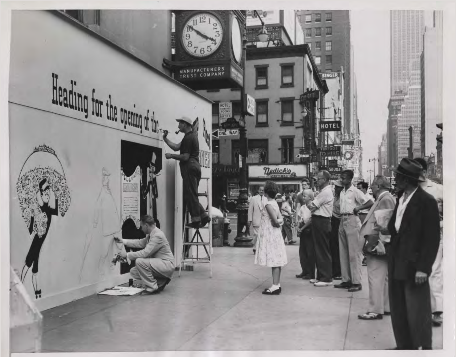
Workers letter and illustrate the construction inclosure for the Lamp Post Corner by hand. The man on the ladder enjoys his pipe while the man below is just trying to keep his suit clean. The Manufacturer's Trust Company clock can be seen near the top of the photo.
