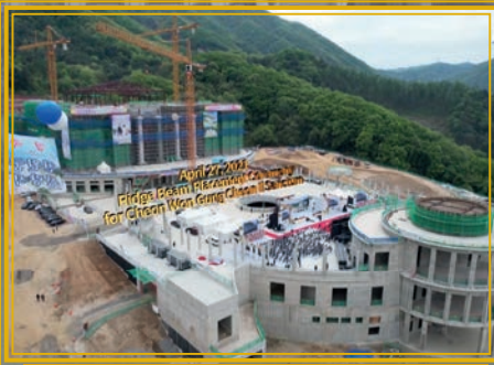
Ridge Beam Placement, April 2021
