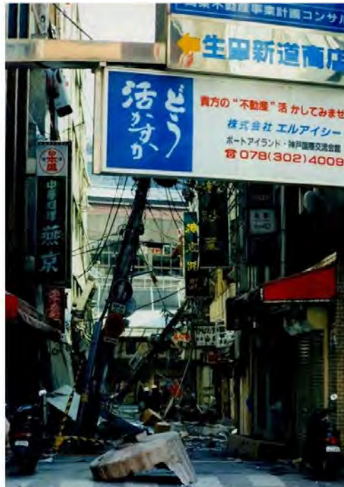
From the Great Hanshin-Awaji Earthquake. Photo (17th January 1995): Akiyoshi's Room / Wikimedia Commons. Public domain image.
