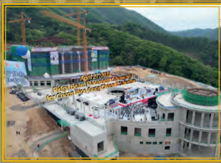
Ridge Beam Placement, April 2021
