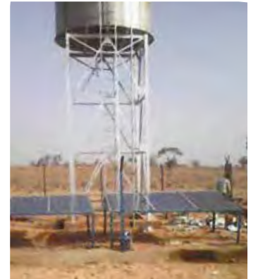
Water Tower with Solar Panels
