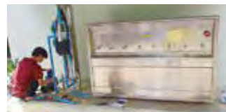
Installed Water Purifier and Water Fetching Place
