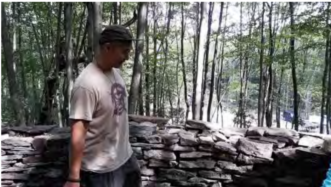
In the Tower being constructed above True Parents Memorial
