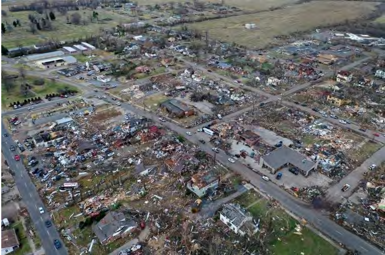
Recent tornado damage in Kentucky (Photo courtesy of NBC News)
