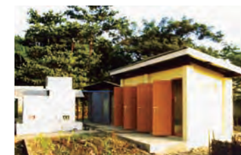
Toilet constructed in Thingun kyun
