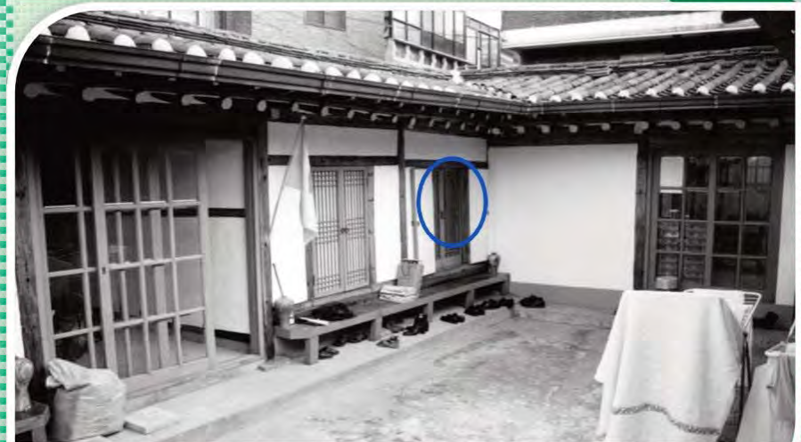
One of the room's at True Father's lodging house was Lee Ki-bong's house
