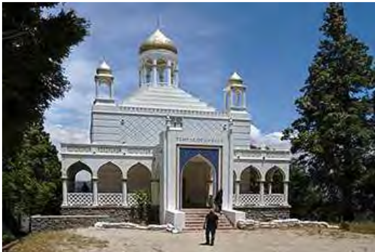
Camp Mozumdar is located in California and is in close proximity to Las Vegas.
