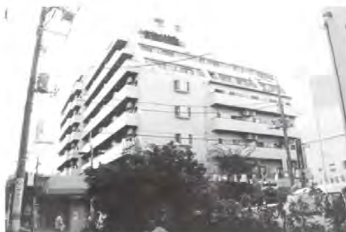
An apartment block in Ogikubo, Tokyo where Hirohisa Koide was forcibly detained in 1992. Photo: Hirohisa Koide
