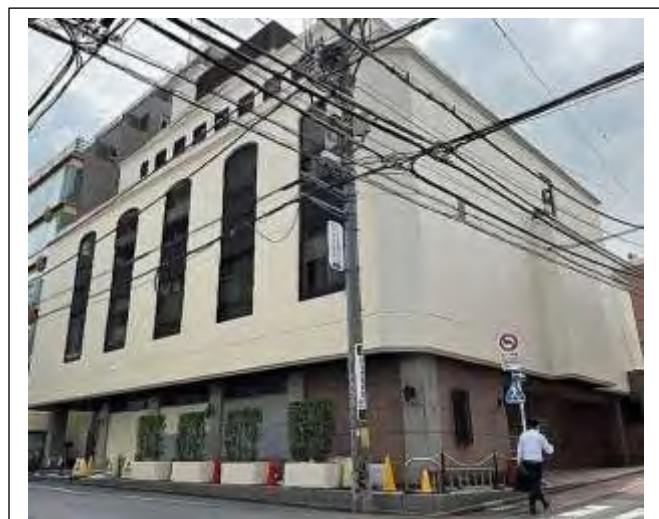
One of 400 facilities nationwide targeted by liquidators: The headquarters building of the Family Federation in Japan, located in Shibuya, Tokyo
