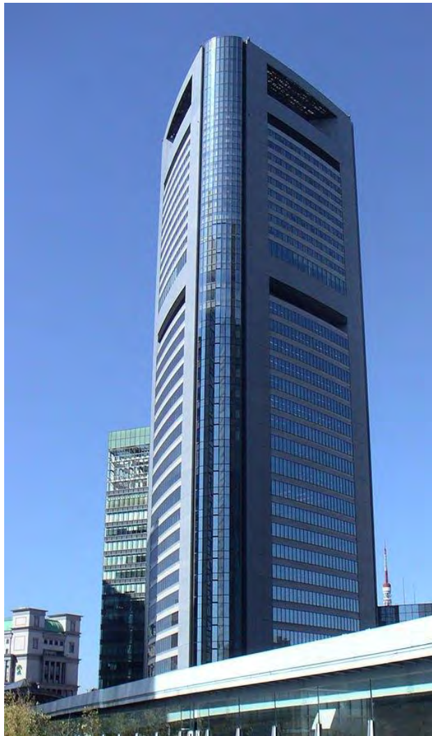
Shidome Media Tower, located in Shiodome, Minato, Tokyo, Japan. Floors 1 - 24 are the headquarters of Kyodo News, Japan's largest news agency
