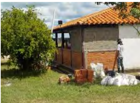
Left: Building a warehouse next to the office
