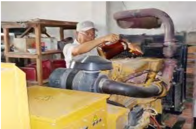
Left: Mr. Nakamura is changing the oil for the generator
