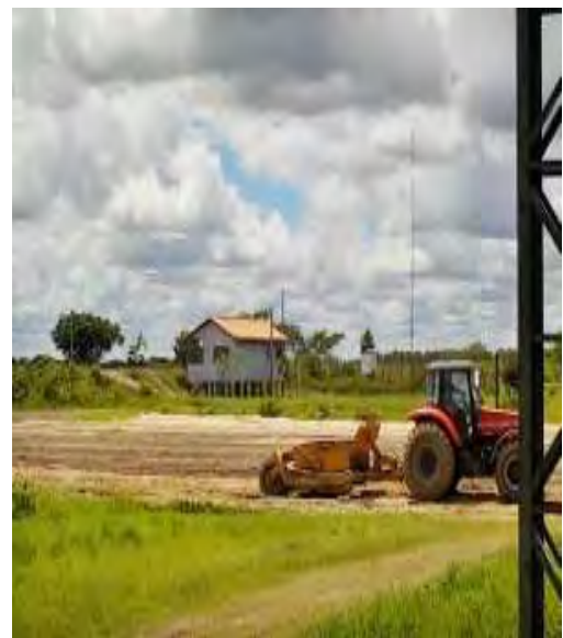
Right: The tractor is working to build factories and residential areas
