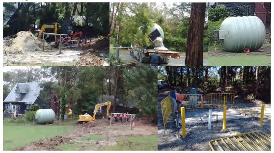
South East Water has now installed and connected the sewerage tank that will pump waste out of the property. The final connections will be made in the coming weeks, completing the project.
