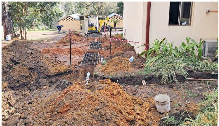
Sewerage connection has now reached the Hall Kitchen, connecting up the 2 grease traps that have been fitted months previous. With this stage coming to a conclusion we look forward to cleaning up the area and beautifying it. The cottage and pastor house are the last buildings needing connection.
