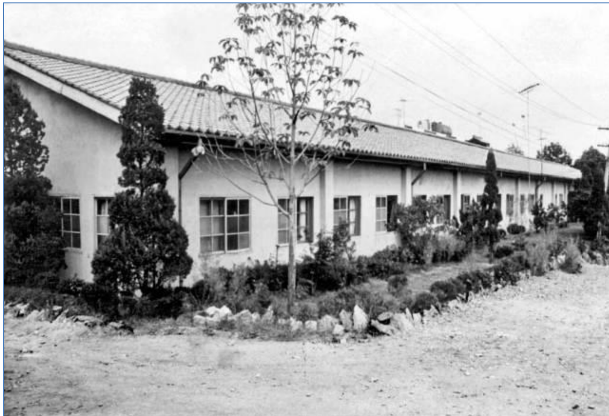
One of three original main buildings of the Central Training Center; two of the three are still in use today
